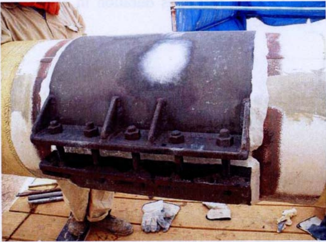
18" Clamp Fully Encapsulated using Aquawrap Composite Repair Systems in Nimr, Oman
