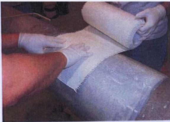
Figure 6 - First layer of Aqua Wrap installed on pipe
