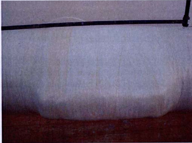
18" Clamp Fully Encapsulated using Aquawrap Composite Repair Systems in Nimr, Oman
