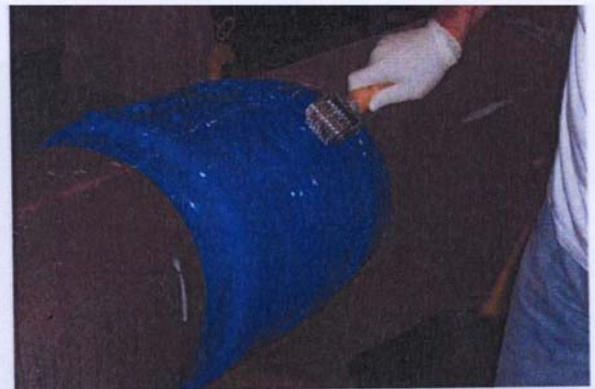
Figure 8 - Perforating plastic wrap to permit off-gassing during cure
